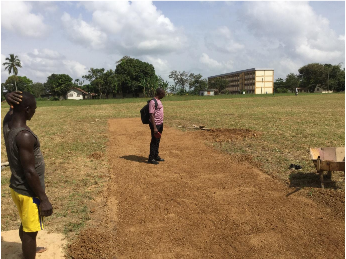
NJALA UNIVERSITY CRICKET GROUND TURF PITCH UNDER CONSTRUCTION
