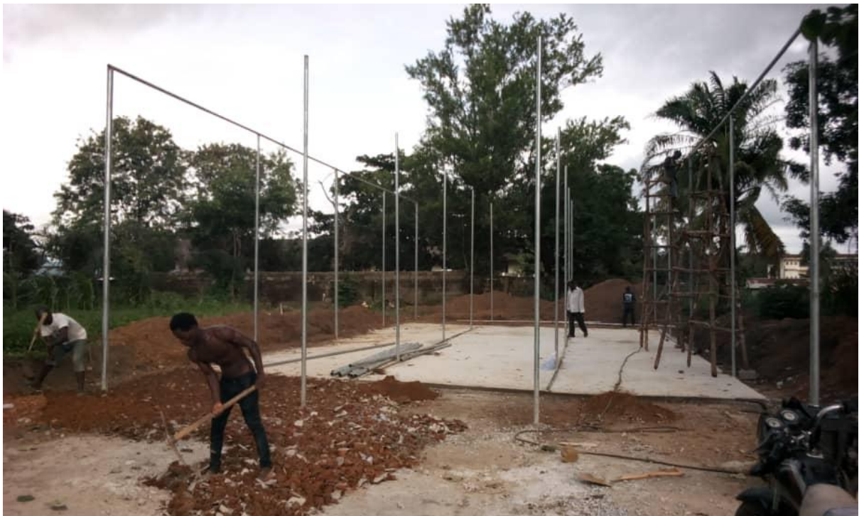
GOVERNMENT SECONDARY SCHOOL BO PRACTICING NETS UNDER CONSTRUCTION
