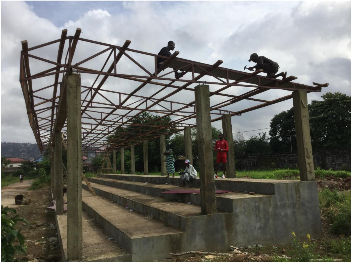
PRINCE OF WALES SCHOOL CRICKET GROUND PAVILION UNDER CONSTRUCTION
